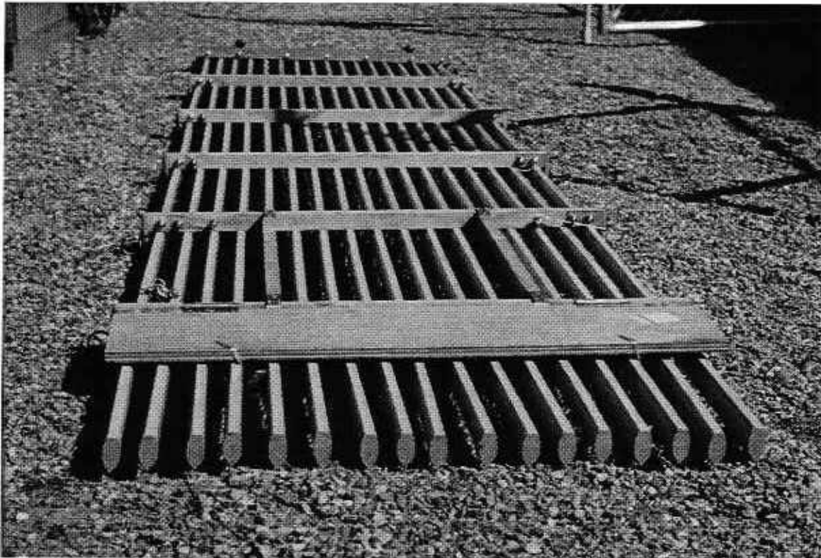
Appendix Figure A-10. Underside of a floating weir panel showing resistant board in the foreground (without extra flotation) and wood framing, Aberdeen Hatchery, Washington.
