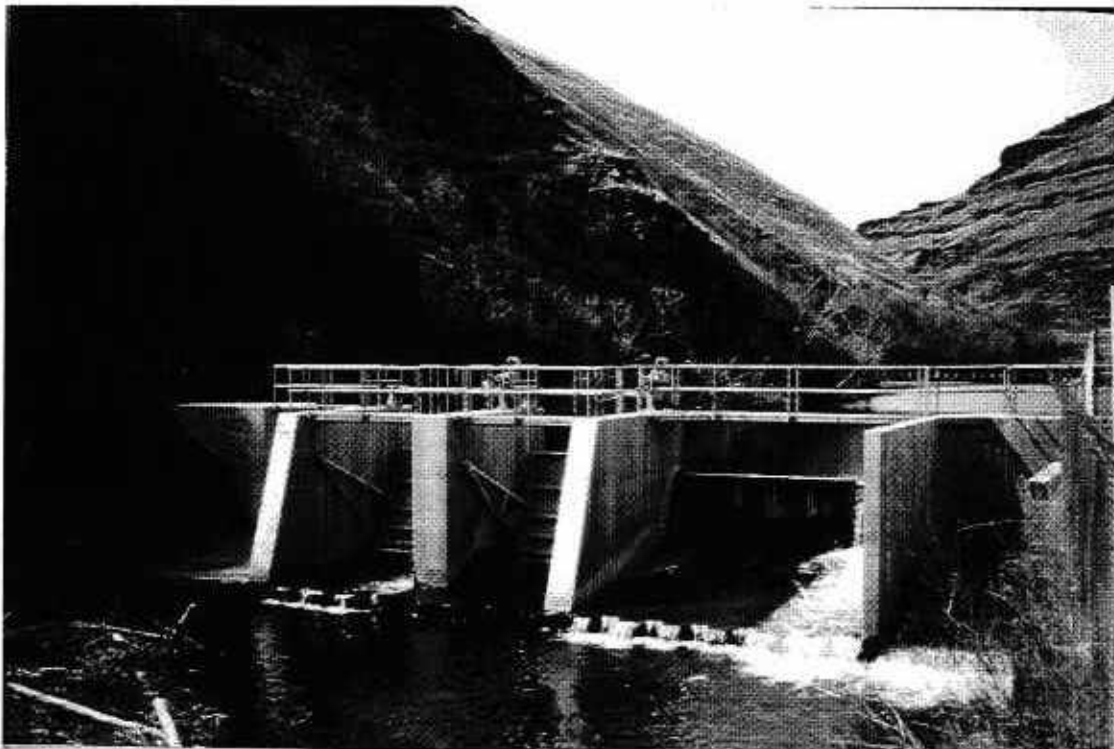
Figure 16. Radial arm dam and velocity barrier used to divert steelhead into adult steelhead trap, Little Sheep Creek (Imnaha River), Oregon.
