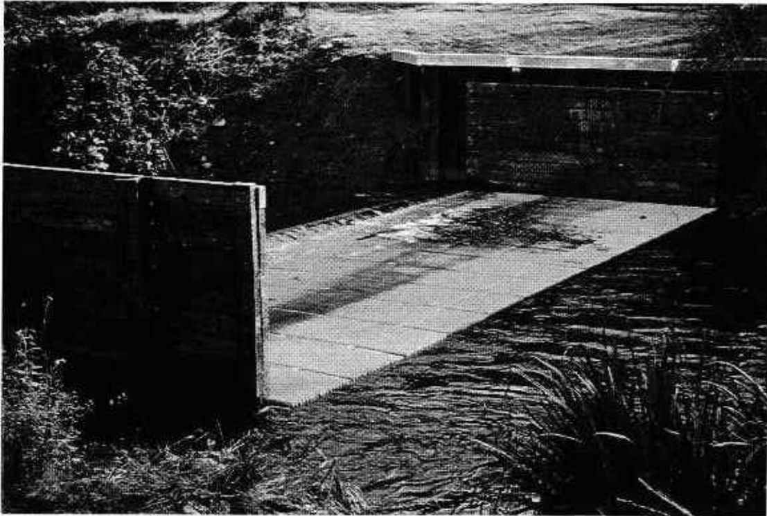
Figure 12. A floating weir at Aberdeen Hatchery, Washington, used to capture adult salmon and steelhead, 1992.
