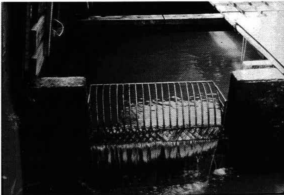
Figure 6. Finger weir in an adult fish trap in a fishway step, Powerdale Dam, Hood River, Oregon.
