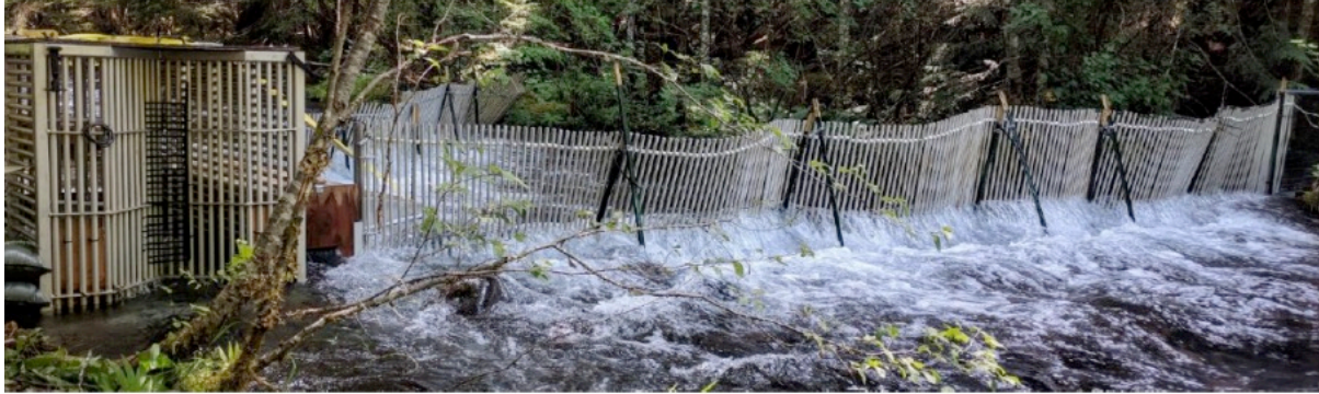
Weir and trap, Pinhead Creek, Clackamas River Basin, Oregon
