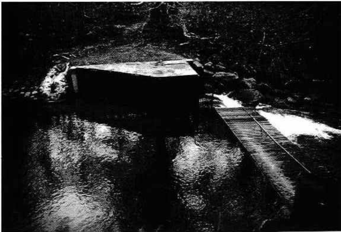
Figure 3. Adult steelhead trap at a horizontal picket weir on Whittaker Creek (Siuslaw River), Oregon, 1992.
